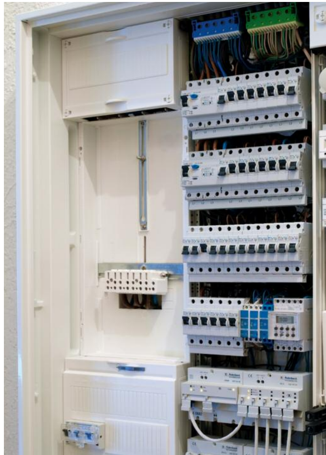
New installation in the electrical distribution box...
